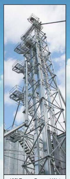
105' Tower: Dry and Wet Elevators Inside Tower and Service Stairway Option
