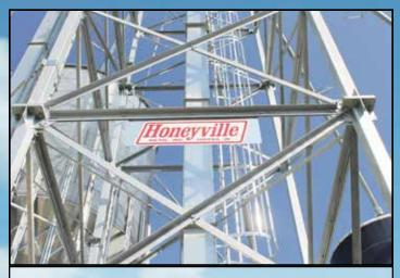
125' Tower: Dry Elevator Inside, Wet Elevator Outside and Service Ladder on Elevator
