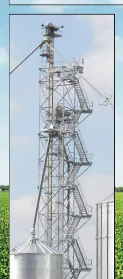
Service Stairway and Custom Walkways to Varying Height Elevator Platforms
