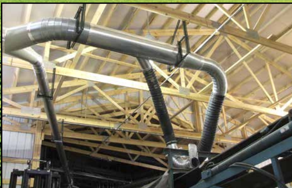
Dust collection on a belt conveyor loading containers with grain. See filter system in photo on right.
