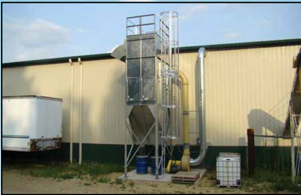
Honeyville EFM Baghouse Filter pulling dust off of the weigh buggies pictured to the right as well as a mixer.
