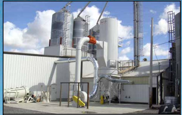
Honeyville MPC Baghouse Filter located in a feed ingredients plant, gathering dust from a truck loadout bay and U-trough augers.
