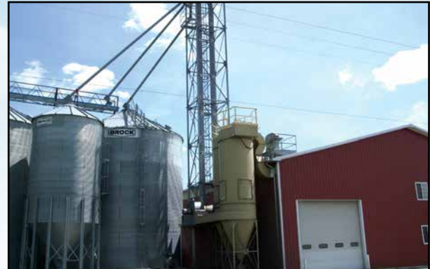
(2) Honeyville EFR Baghouse Filters located at a large farm seed cleaning operation.
