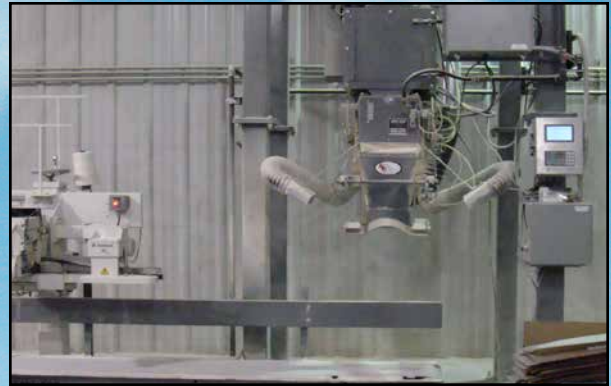
Bagging station in a nutritional plant, with (2) 3" suction lines to pull dust away from the fill station.
