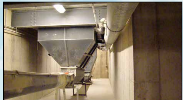
Semi unloading pit hopper and rail car pit with suction pipe connections. View from bottom side of the pit.
