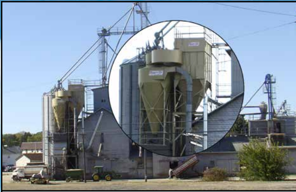
Honeyville MH Series Cyclones shown with an EFM Baghouse Filter, pulling dust from various locations in a country feed mill.
