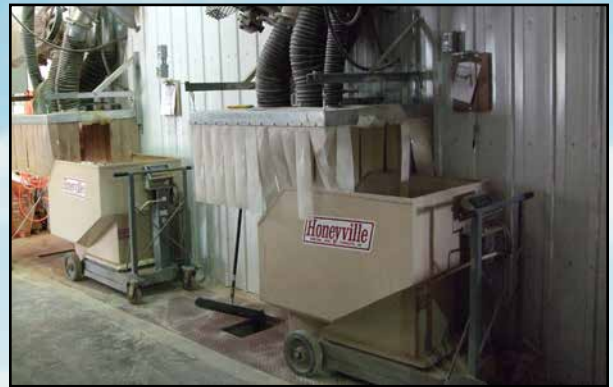
Suction hoods for a Honeyville Weigh Buggy fill station at a feed mill. This equipment is related to the photo on the left.
