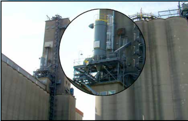
Honeyville EFR Baghouse Filter on top of a concrete silo pulling dust off of various locations.
