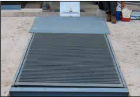
Drive-over pit hopper with bar grate provided in 12" wide lift-out sections for easy access
