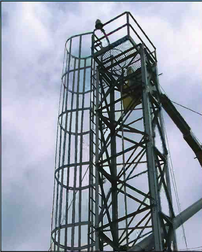
46" x 24" 4-Leg tower with ladder, safety cage and service platform
