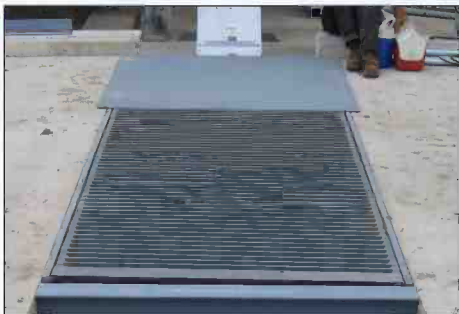
Drive over bar grates for pit hoppers
