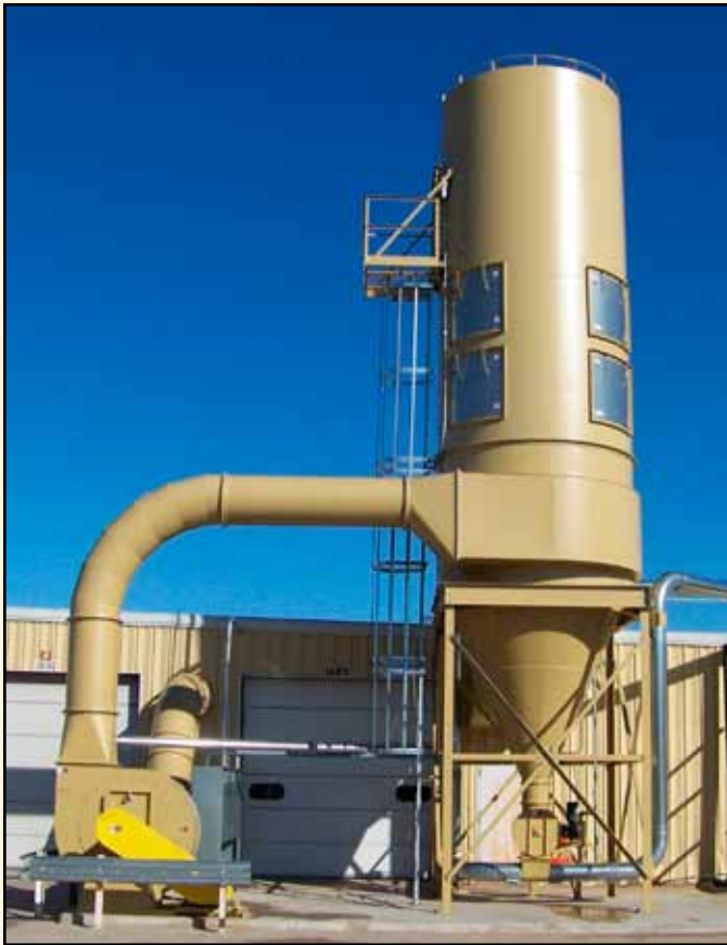
Standard HF series fan with a medium pressure pulse cleaning baghouse filter.
