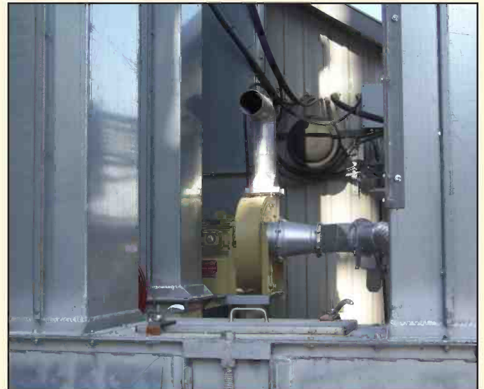
6" direct drive fan in an agriculture application. This fan is pulling dust off of (2) grain bucket elevators.
